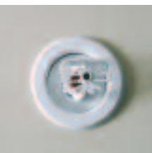
Sidewall Sprinkler
